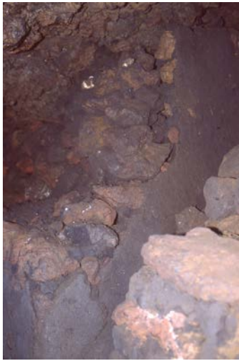
Figure 9.4. Second Narrowing south side, even application of concrete to ends of middle section: a. (left) facing southeast, west end (photo by Sload 1978); and b. (right) facing southwest, east end (photo by Sload 1978, © R. Millon).
