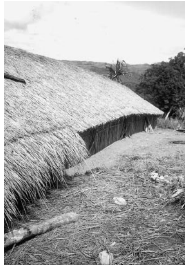
FIGURE 4 Thatching in completion. A part remains to be trimmed at the edges
