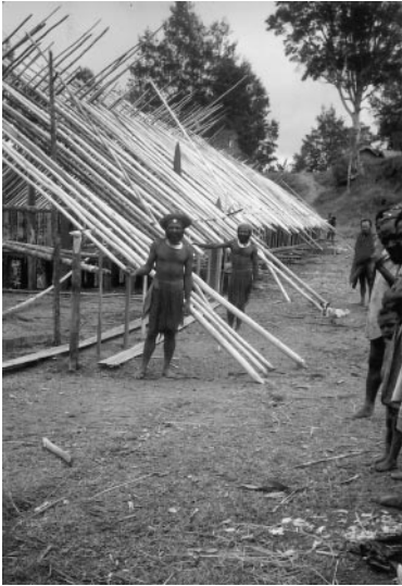
FIGURE 1 Placement of the rafters at early stage of construction
