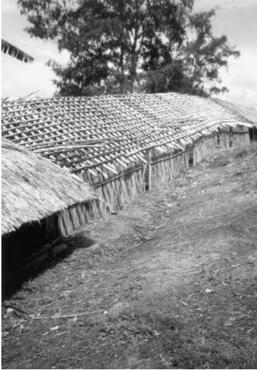
FIGURE 3 External view of rafters and roof cross-pieces after trimming, and part-thatching of roof
