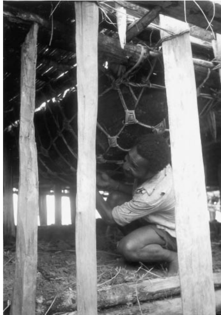
FIGURE 6 Lashing together the lianas (ropes) holding the firebox in a residential cell of the longhouse. Each man or pair of men, or men with families, would cook on a separate fire made in this way
