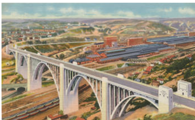
The iconic Westinghouse Bridge, (WQED 2008)
